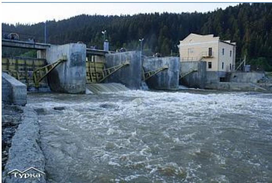
Yavirska small HPP- 450 KW
